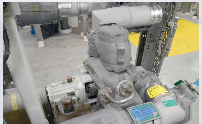
Finder hot water circulation pump. It is sealed with a single seal type H75VN/50-E87-A4-OR. Supply in accordance with API Plan 11.
