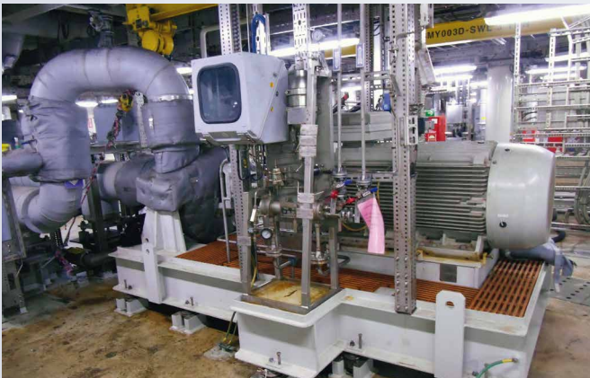
Finder circulation pump for heat carrying medium sealed with H75FD/90-E3-A1 double seals, supply in accordance with API Plan 53B.
