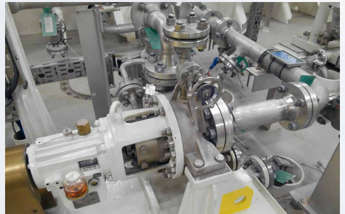
Finder drinking water pump with single seal H75VN/50-E93-A1, supplied in accordance with API Plan 11.
